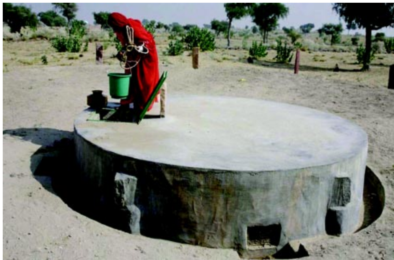
Drought proofing by building water tanks
