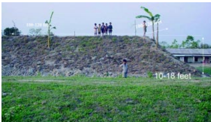
Raised earth-work flood shelter
