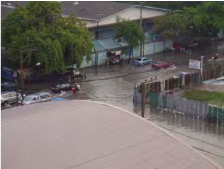
Flooding in Bangkok
