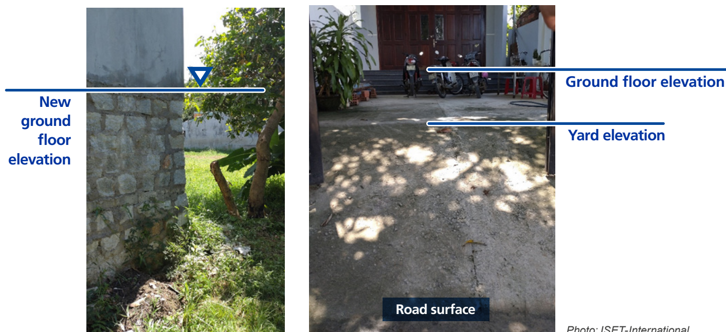
Figure 5 Images of houses in Nhon Phu after repeated raising of ground elevation
