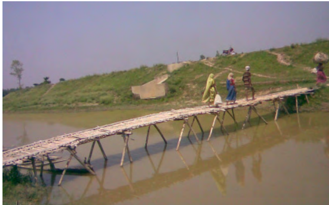
Temporary bridge in Nepal Tarai
