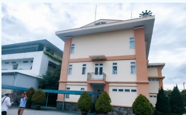
(Top) A high-powered warning system being installed in Hue City, Vietnam © Hue City DRM Office. (Bottom) A high-power siren located in the north of Hue City © ISET Vietnam Office
