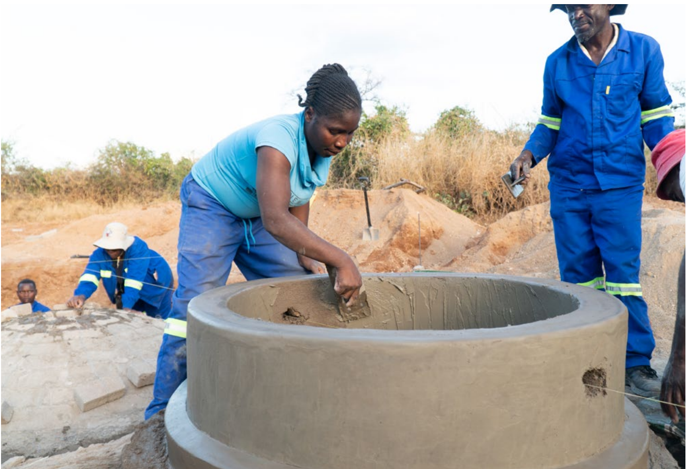
Evidence Mutitsve, one of the three women trained in the construction of biogas digesters © Practical Action Zimbabwe
