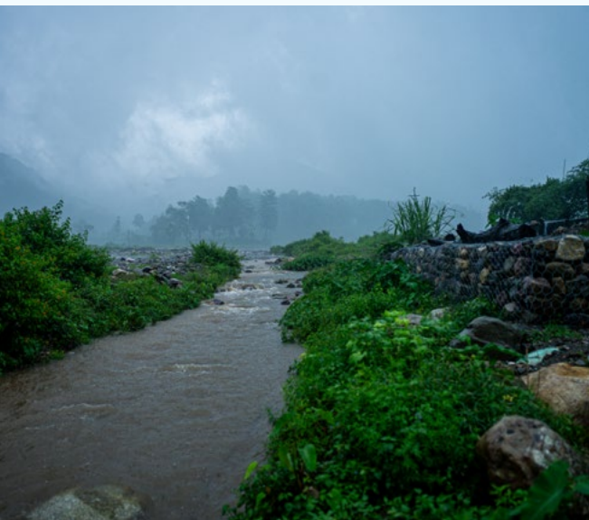
The gabion wall constructed within the riverbed in Chiran, Kalakot community of Alital rural municipality, Dadeldhura, plays a vital role in shielding water pipes and protecting the community from floodwaters © Mercy Corps Nepal
