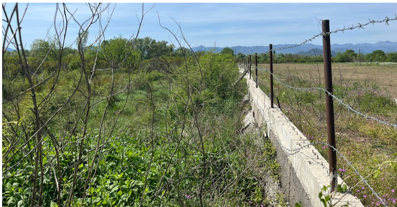
The flood protection wall in the community of Ponari was rehabilitated by the Red Cross of Montenegro together with the Zeta Municipality to mitigate impacts on livelihoods © Red Cross of Montenegro
