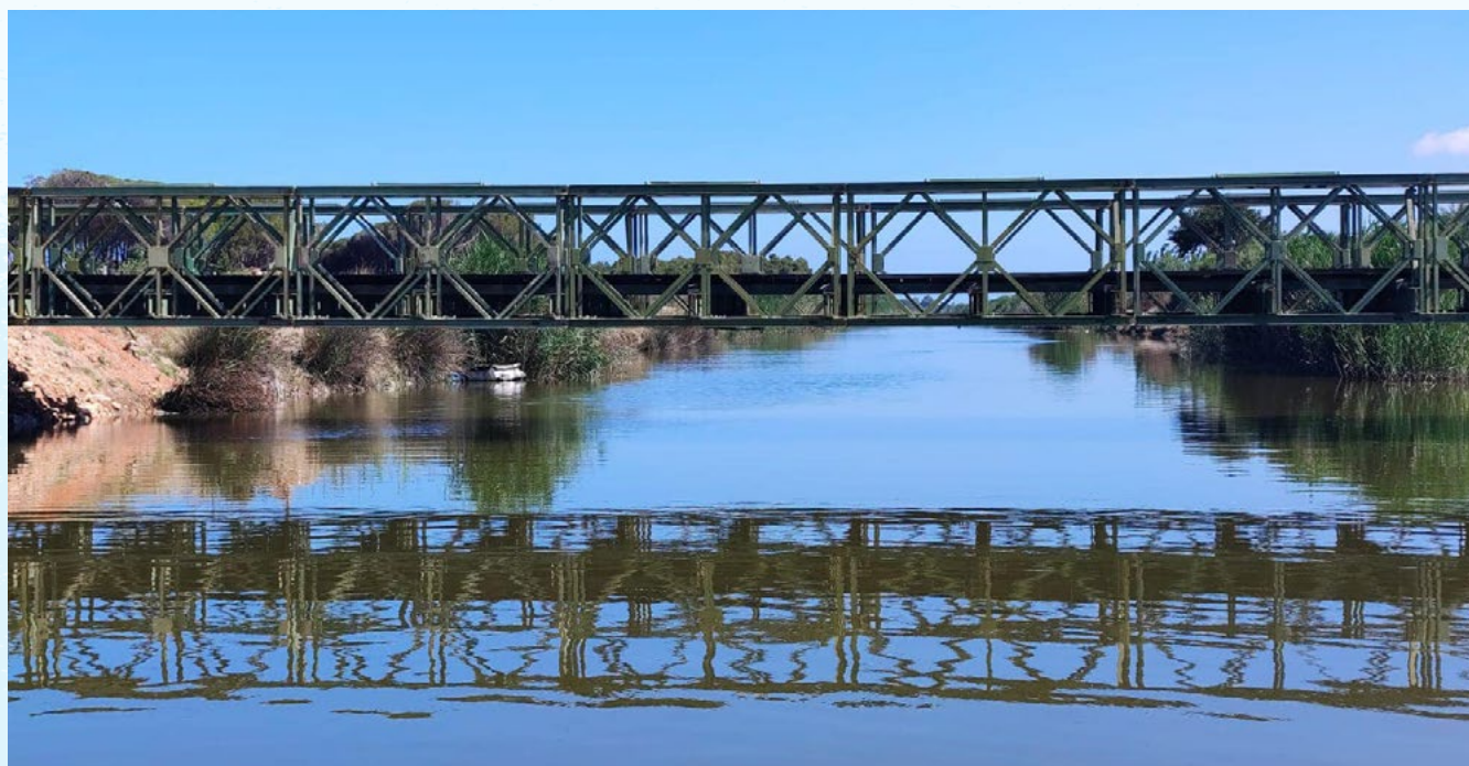
New, fortified bridge in the community of Darëzezë to support evacuation during floods © Albanian Red Cross
